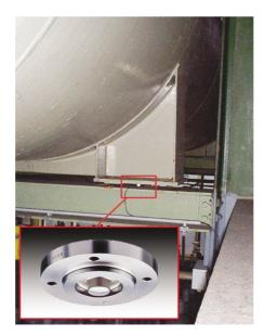
Due to the gravimetric measuring principle the accuracy is totally unaffected by the product in the vessel. Whether liquids or solids, whether dust or foam- the sensors reliably indicate the correct content. As the sensors are not in contact with the product this method completely avoids any contamination of the vessel contents or mechanical or chemical abrasion of the sensors by the product.
